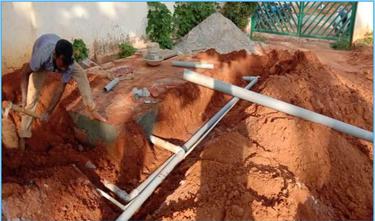
Fig: Underground Sump in Construction Phase
